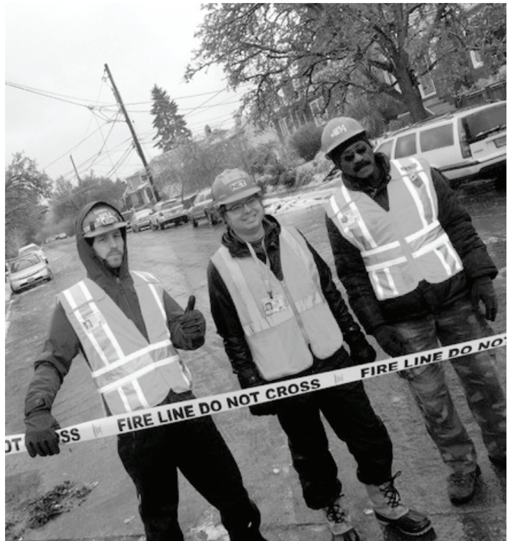
Three NE Portland NETs, including Woodlawn Assistant TL Brendan Dunn, securing the site of a downed power line. Photo by Ethan Jewett.
