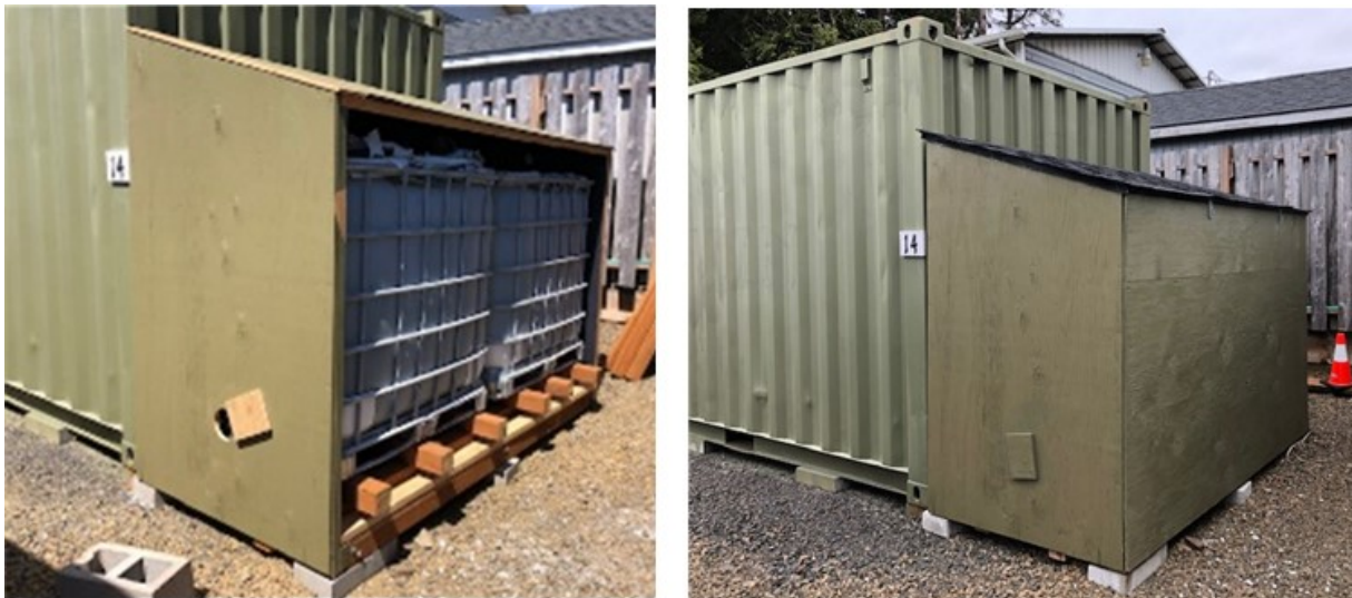
Figure 46: Two 275-gallon Caged Water Containers. Left: shed during construction. Right: finished shed.
