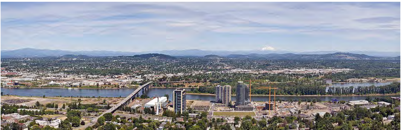
Figure 7. Looking toward East Portland showing buttes in background and regular geometry of city streets in foreground (Image courtesy of wikimedia).
